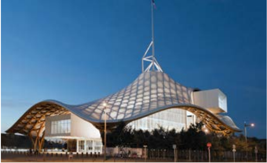
Centre Pompidou Metz
